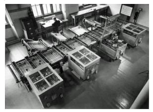
The Differential Analyzer weighed 100 tons, used 2000 vacuum tubes, thousands of relays, 150 motors, and approximately 200 miles of wire.
