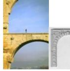
Beginning in the 4<sup>th</sup> century B.C., Romans constructed huge aqueducts to carry water for distances up to 50 miles. These structure were built on continuious gradual declines to transport water by forces of gravity. On the Pont du Gard aqueduct, which carries 100 gallons of water a day for each inhabitant of the city, each large arch spanned 82 feet.
